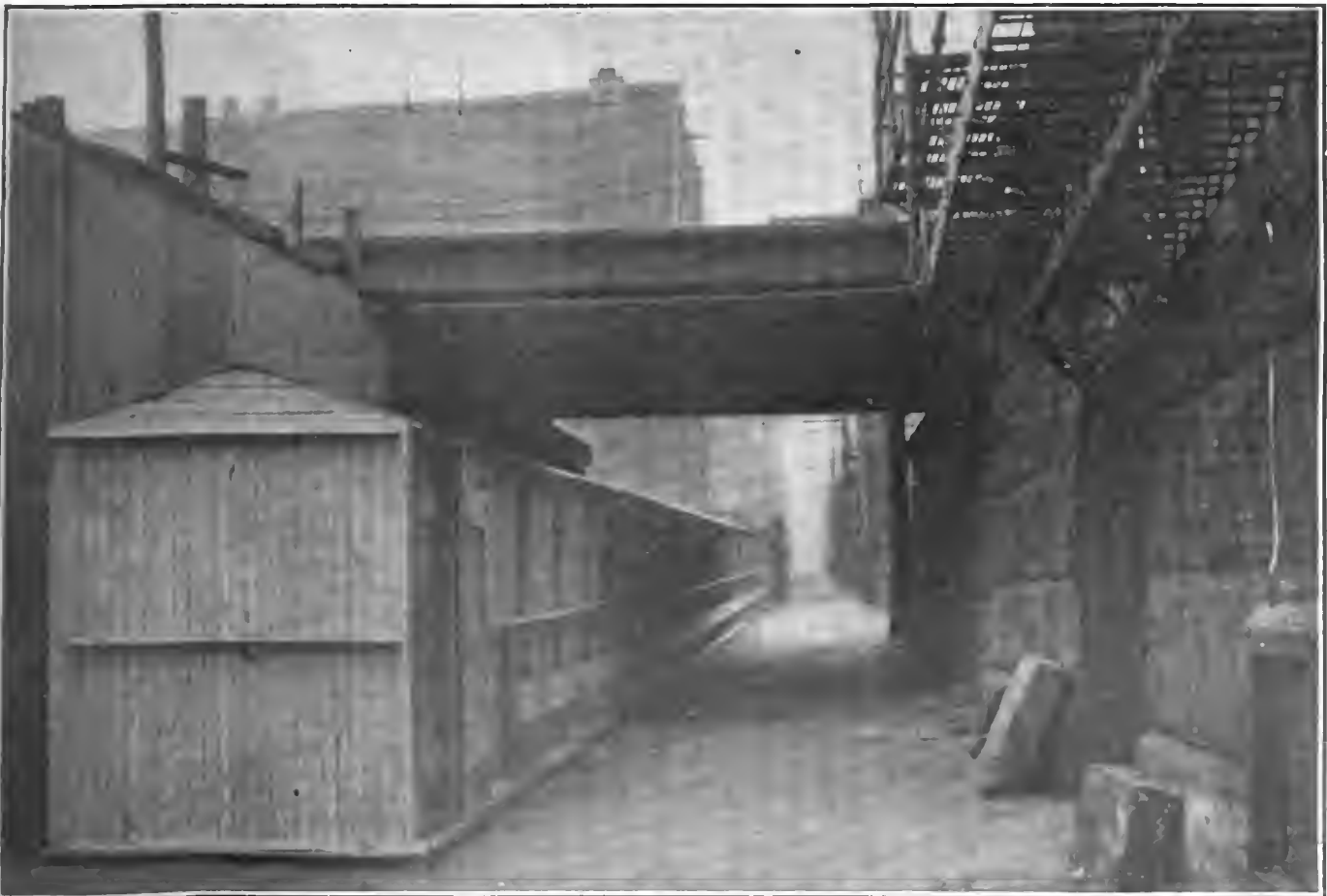
SIX-FOOT COVERED PASSAGE, 300 FEET LONG, CONNECTING REAR ENTRANCES OF THE COLISEUM AND ARMORY, ERECTED ESPECIALLY FOR THE OCCASION OF THE PRESENT AUTOMOBILE SHOW, FEBRUARY 3 TO 10.
